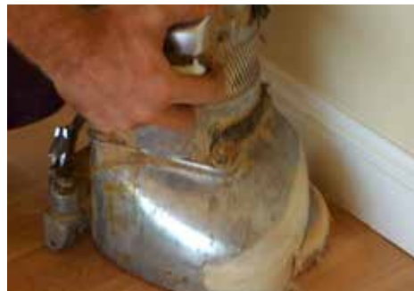
Edge sanding requires a smooth action to blend into the floor.
