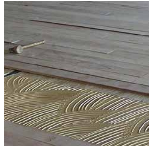
Adhesive spread prior to fixing
