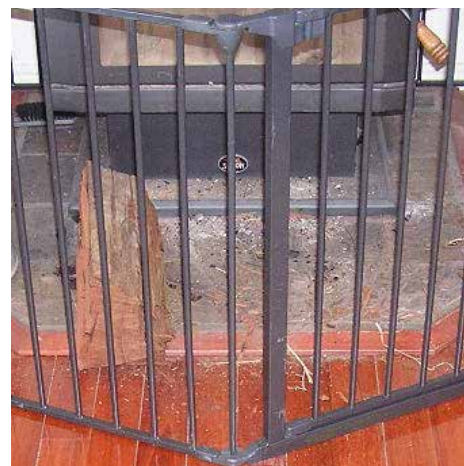
Intense heating sources can cause localised shrinkage.
