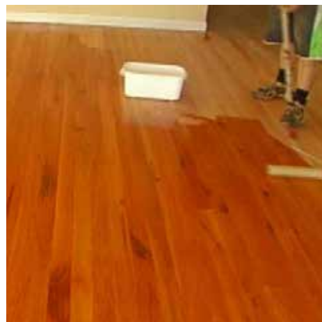
Application of the initial coat.
