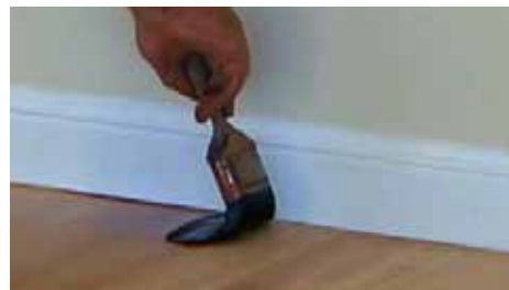
Cutting in the finish around perimeter walls.
