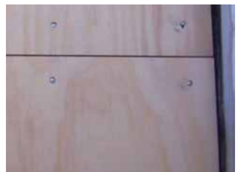
Fixing of the plywood subfloor through the polyethylene membrane and into the slab.
