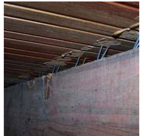
Buckling of 80 mm wide Spotted Gum boards secretly fixed to pine joists in a humid locality.
