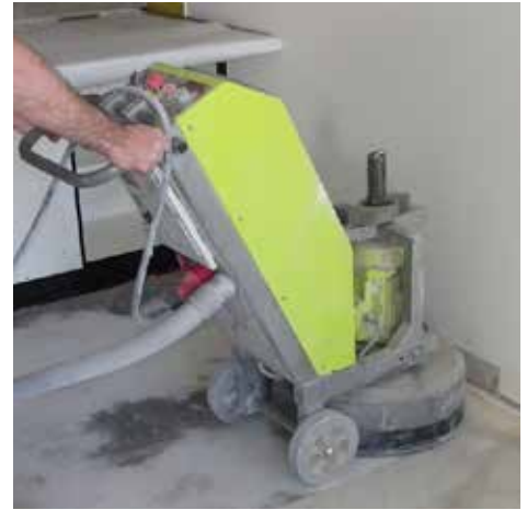
A slab being ground flat and also removes contaminants
