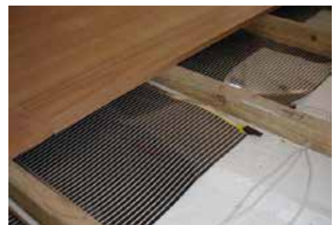
Blackbutt flooring (130 mm wide) with electric underfloor heating in Adelaide
