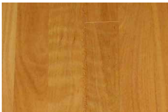
Cork intermediate expansion joints blend in well with timber floors.
