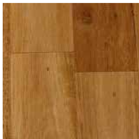
Boards ends should be spaced out and preferably 450 mm or more apart.
