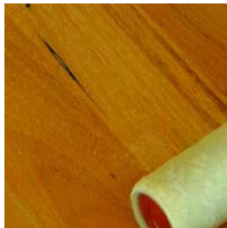
Application of the second coat.
