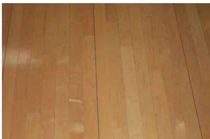
Particularly for wide floors or in moist climates small regular gaps can be used to provide the additional expansion allowance needed. These often close during humid periods.
