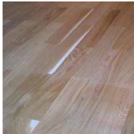
Imported product where their grading rules permit the light coloured sapwood. As this is infrequent it is prudent to check that this meets client expectations.
