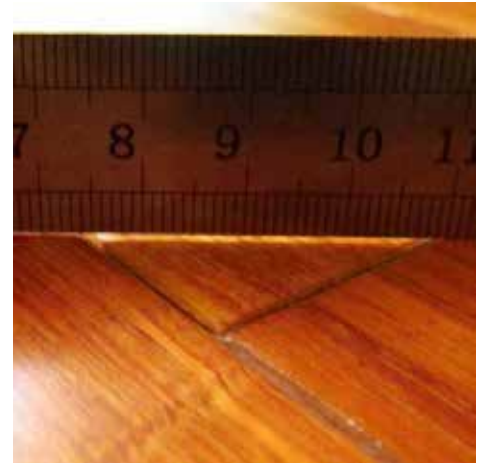
The effect of beveled edges minimising mismatch effects
