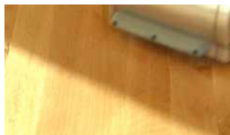
Second pass of sanding at 45° to board direction.
