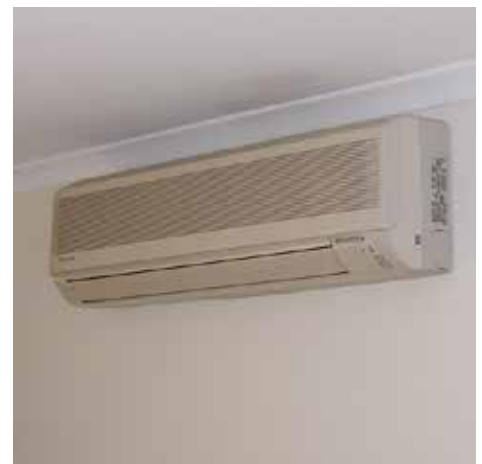
In warm climates these units are referred to as reverse cycle split system refrigerative air conditioners. In cold climates like New Zealand they are referred to as heat pumps.
