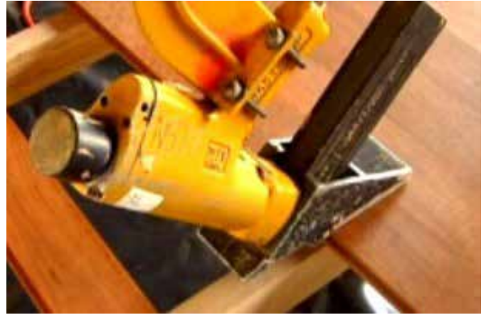
Secret fixing is recommended for boards up to 85 mm in cover width.
