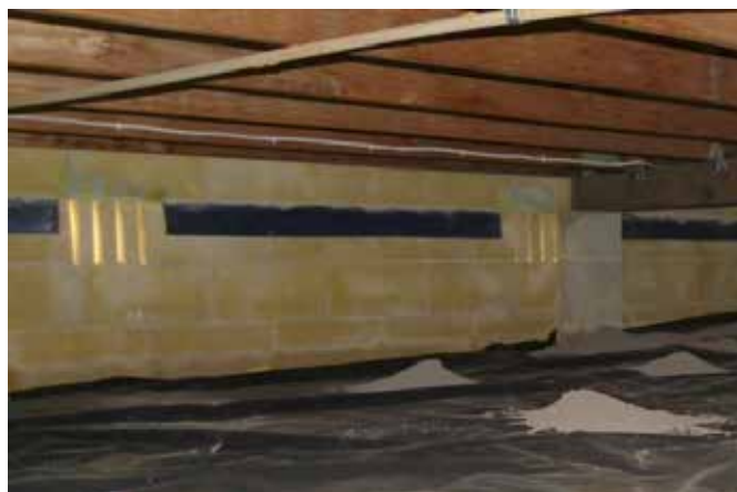
With frequently damp soil conditions the subfloor ground level was raised with crusher dust and a polyethylene membrane laid over it
