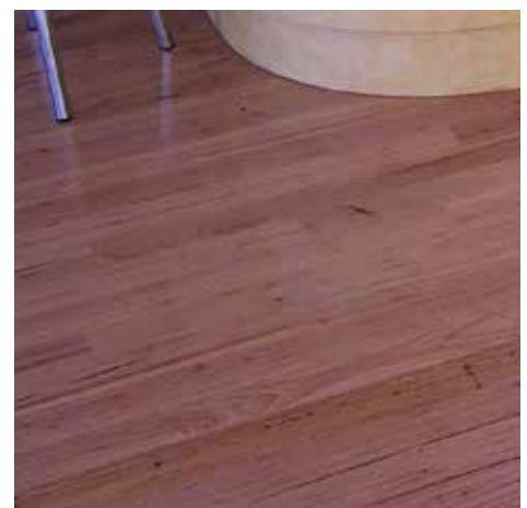
Direct adhesive fixed 80 x19 mm Standard Grade Blackbutt
