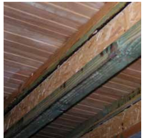
Timber floors are successfully laid over a range of solid timber and engineered joist systems.
