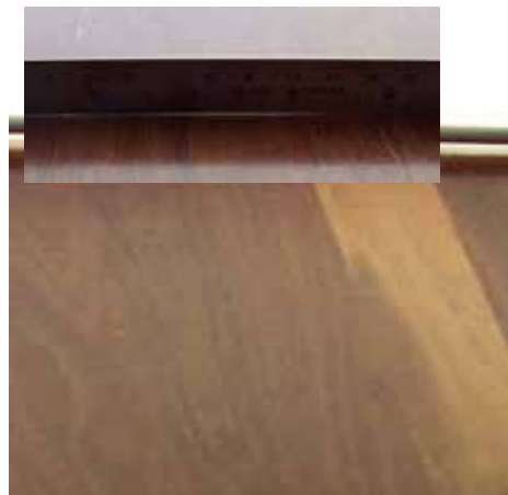
Cupping – Board edges higher than the centre of the board, but which is barely visible in the floor.
