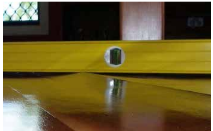
The photo shows possible consequences of not using a slip tongue and not fixing these boards correctly.
